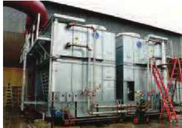
EMSCO's installation expertise extends from civil construction through final system commissioning
