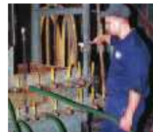
Testing power leads for flow
